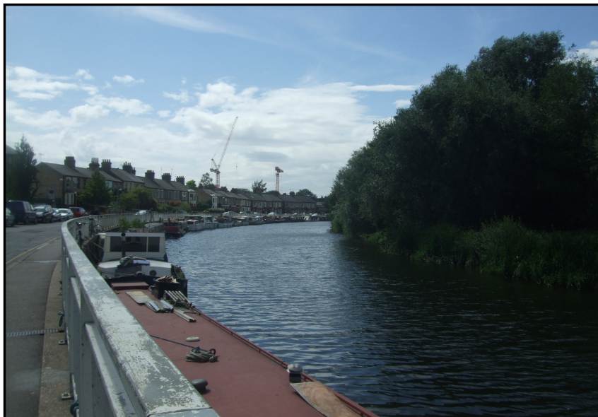
View upstream along a zone of mooring. Mooring zones are currently situated along the banks of Riverside, except for a prohibited zone along the right bank in front of the Museum of Technology. Vegetation encroachment here is limited.
